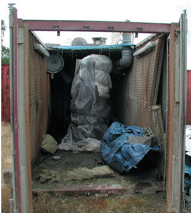
Motorblok in container. © Materials Consult.
